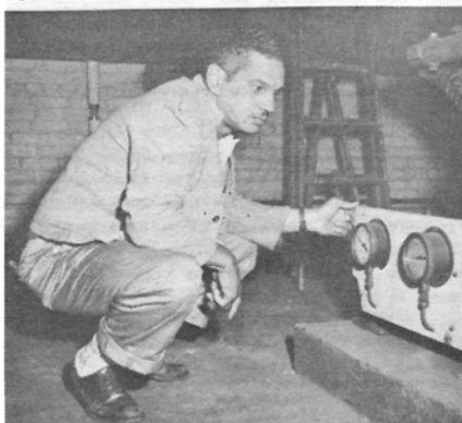
Spencer Russell checks the pressure gauges on one of the compressors that supplies the television studio in Building #2 with cool air.
