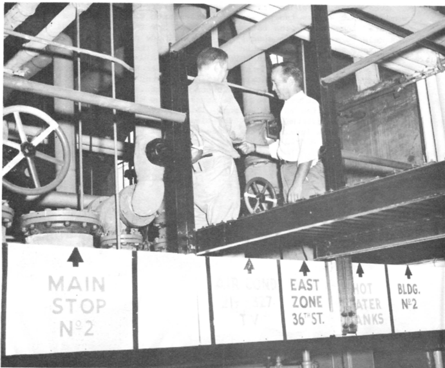
On a catwalk above the boiler in the basement of Building #1, mechanic Jack Gulick receives instructions for operating the motorized and manual valves that control various heating zones from supervisor Herbert Herzog. (Photos by SP4 NORMAN L. MICKEY)
