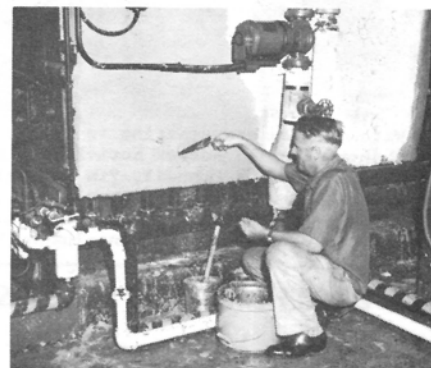
William Reynolds, boiler fireman, recovers a boiler in Building #6 with insulating asbestos.
