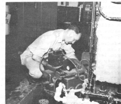
Boiler fireman Ludwig Leib cleans an oil burner so it will be ready for efficient operation.
