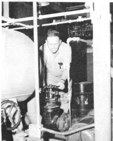
Edward Thoman completes the swing over from one set of vacuum and condensate pumps to another in boiler room of Building #1.
